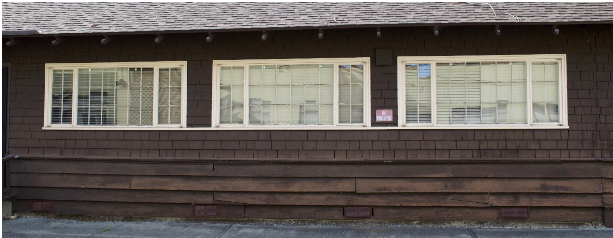
Photo 14 Steel sash windows in addition (1939), looking north
