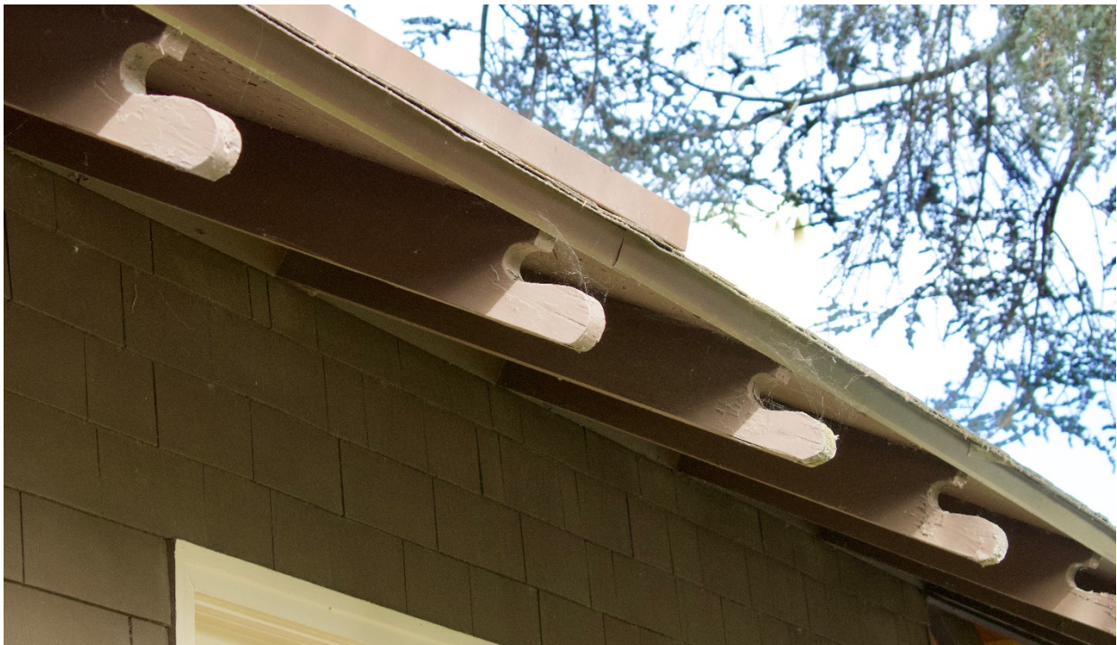
Photo 6 Exposed rafters and rafter ends, looking up
